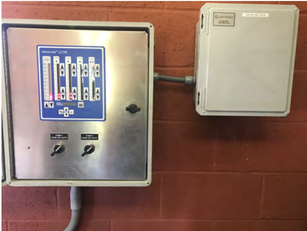
Cattron's Messenger BLE integrated with LC150. RemoteIQ pump monitoring dashboard.
